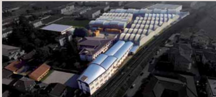
S•CAB sede/headquarters - Coccaglio (BS) Italy
